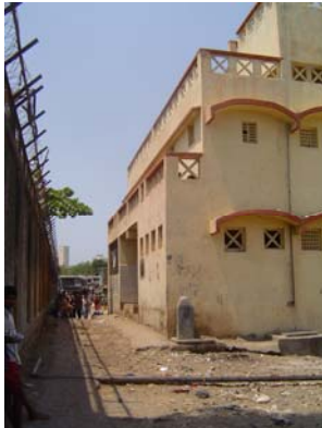
Figure 4: Toilet Block in Ganesh Murti Nagar
