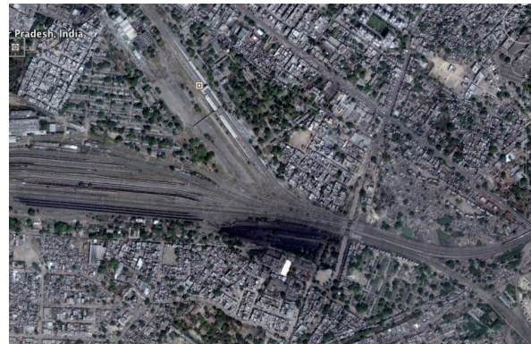
Figure 32: Railways splintered the city during the advent of Industries in India during Colonial Period: Kanpur City
